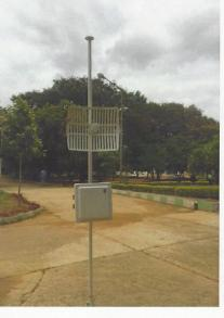
Sabal is a high throughput, high power, exceptionally reliable, modular and effective wireless solution for outdoor use cases. The outdoor Access point (AP) complies with IEEE 802.11ac standard and is backward compatible to IEEE 802.11a/b/g/n standards. The outdoor AP has triple software programmable radios to support 2.4 GHz & 5 GHz concurrent users. It supports a minimum of 2x2 MIMO on both the radios/bands and can be extended up to 4x4.
